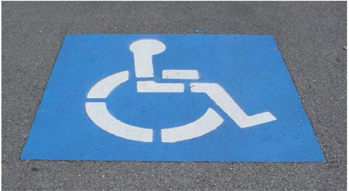
Figure 14 Accessible Space Marking
